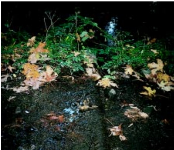
Poor cross drainage has led to erosion and has accelerated trail wear
