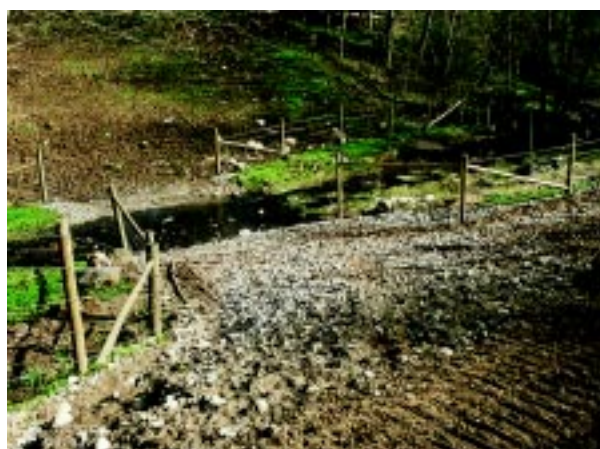
A gravel surfaced crossing allows livestock direct but managed access to stream
