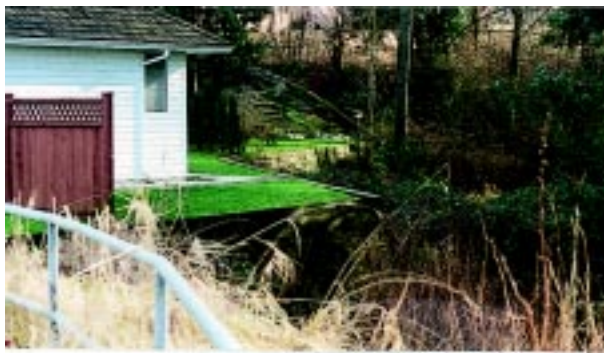
Timber retaining walls with rail fencing can be effective barriers
