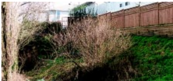
Timber fencing atop a timber retaining wall prevents disturbance of leave area
