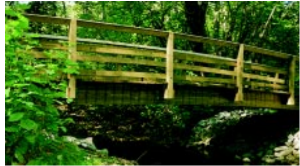
Clear span bridge: footings are located outside the wetted perimeter
