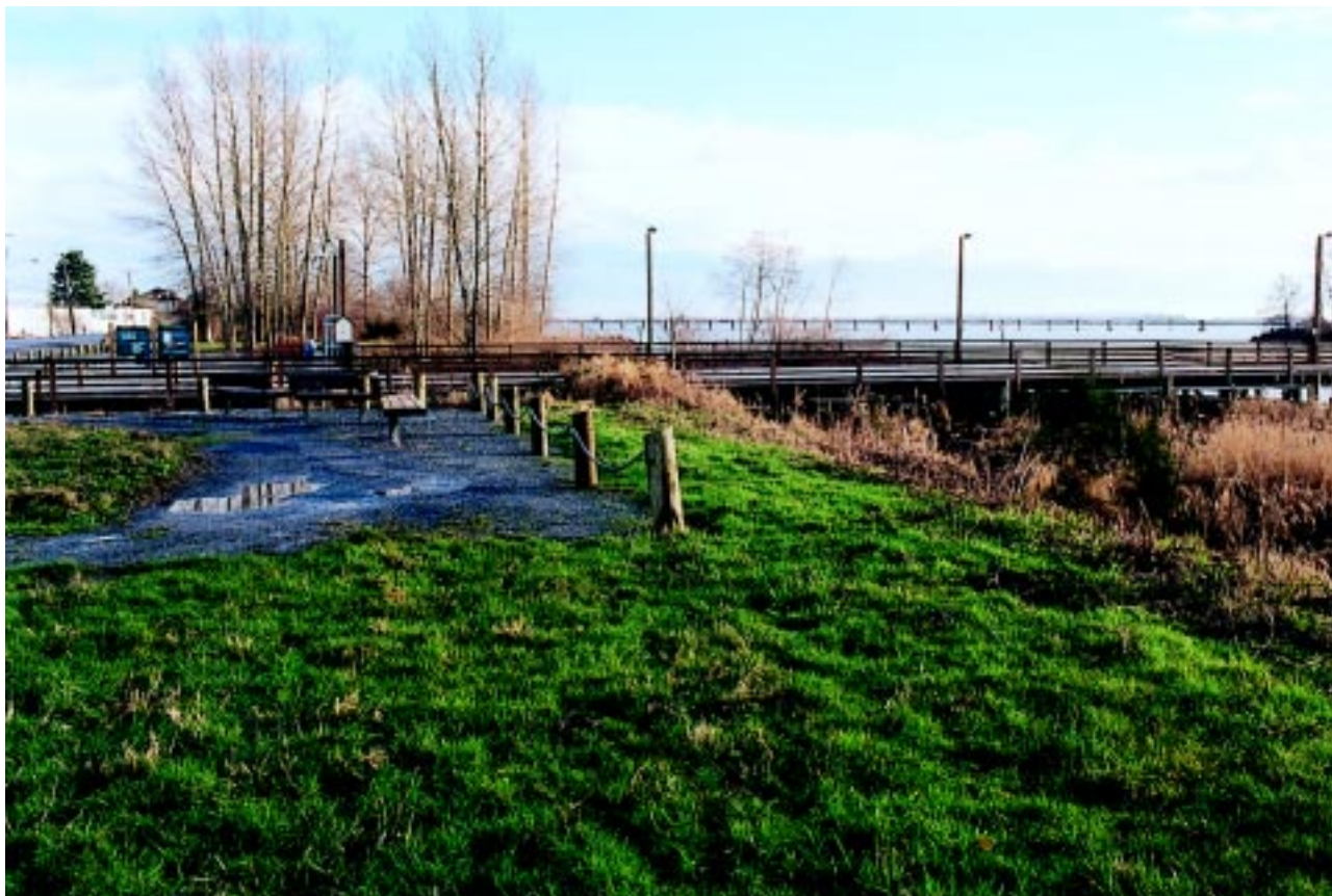
The pier and seating area at London's Landing along the South Dyke Trail in Richmond, B.C.
