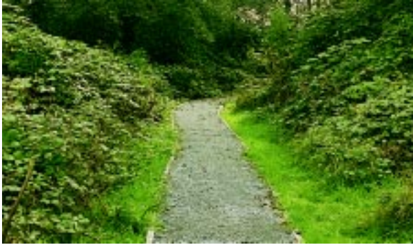
Example of a crushed aggregate path surface
