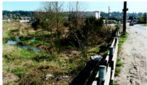
This open fence design is not effective in preventing trespass and litter into the stream
