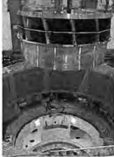
L; Crews replacing damaged concrete in the steep section of the WAC Bennett Dam Spillway Chute. R: The new turbine runner on Unit 3 is lowered into the turbine pit at GM Shrum.
