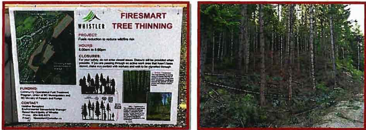
Figure 3. Fuel management treatment in Whistler funded by strategic wildfire prevention initiative - July 2014.
