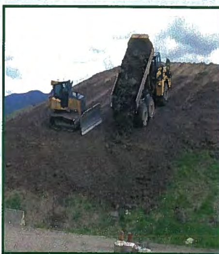
(Equipment working on covering the landfill)
