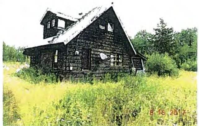
11. Back of Cabin Facing NORTH/EAST
