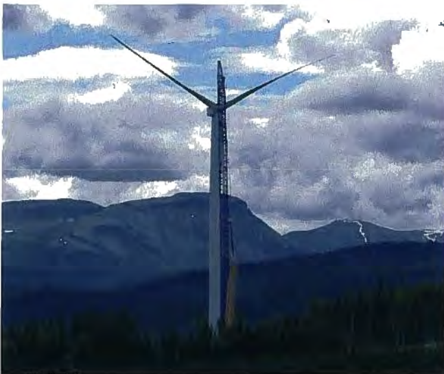
The Meikle Wind Power Project, located near Tumbler Ridge, is B.C.'s largest wind farm with 61 turbines.
