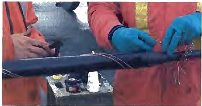
New steel wire armour submarine cable being spliced together.
