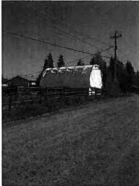
View of accessory building from Sinkut Frontage Road
