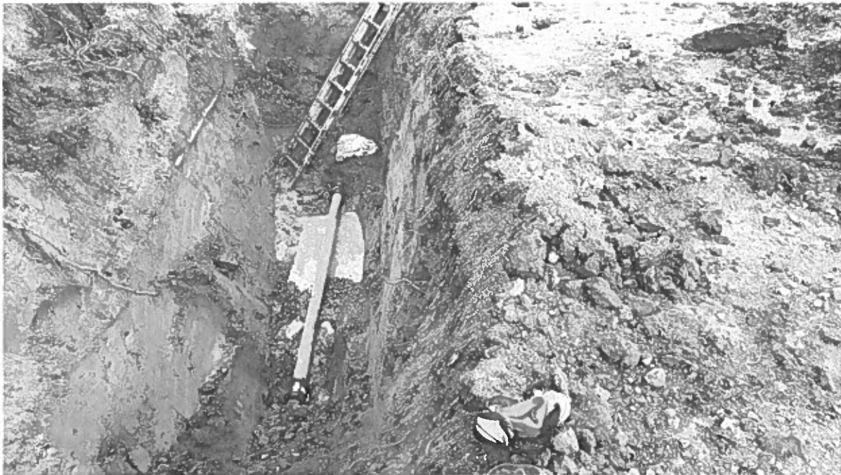
FIGURE 4 – WATERMAIN REPAIR ON CORPORATION STREET
