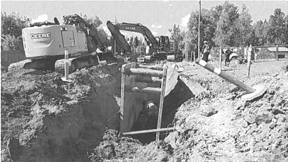
FIGURE 7 – WATERMAIN TRENCH ON ALEXANDRA STREET
