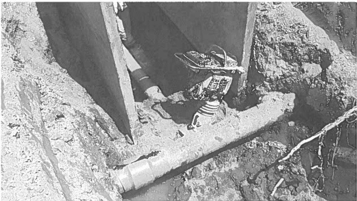
FIGURE 8 – JOINT PROTECTION ON EXISTING SEWER MAIN AND WATER MAIN ON ALEXANDRA STREET
