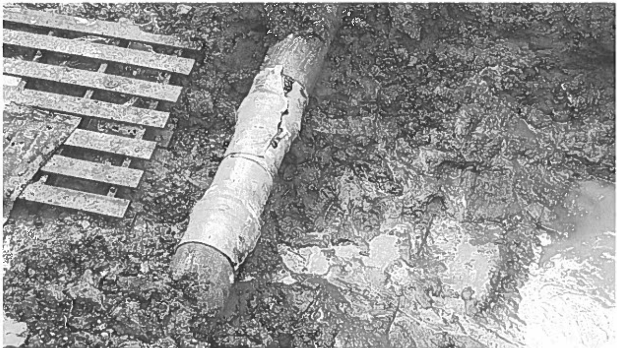
FIGURE 10 – REPAIRED AC SEWER MAIN ON ROYAL STREET
