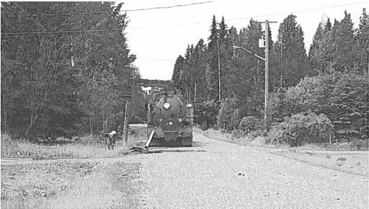
FIGURE 11 – VAC TRUCK LOCATING THE WATERMAIN ON 5 TH AVENUE
