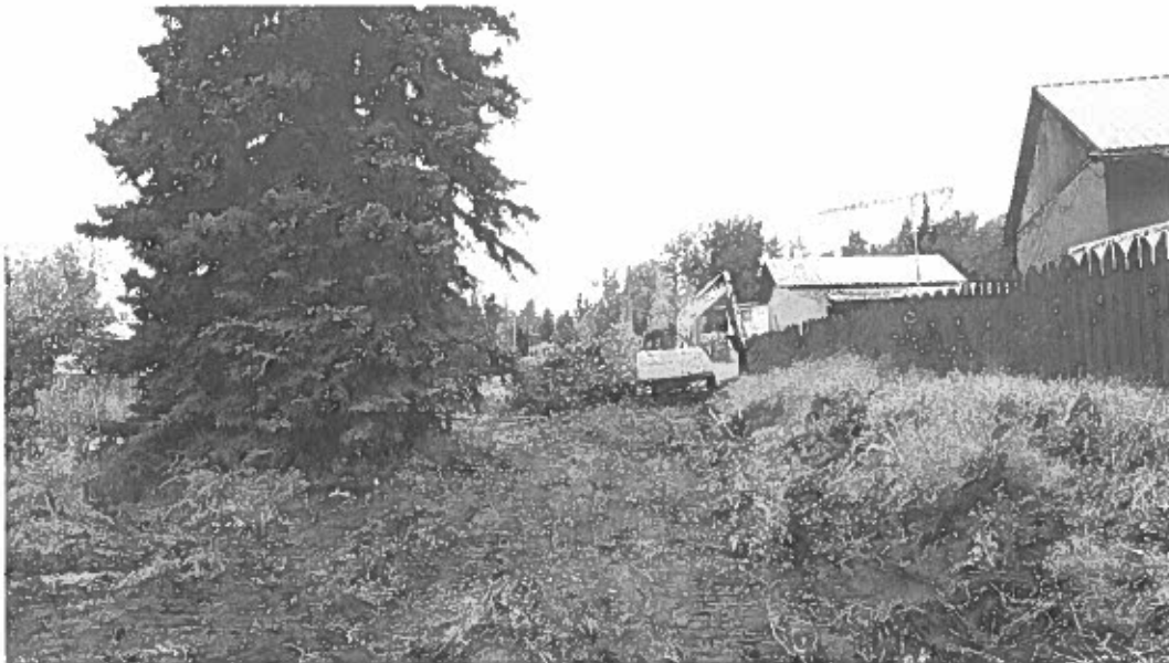
FIGURE 2 – CLEARING AND GRUBBING ON ALEXANDRA STREET
