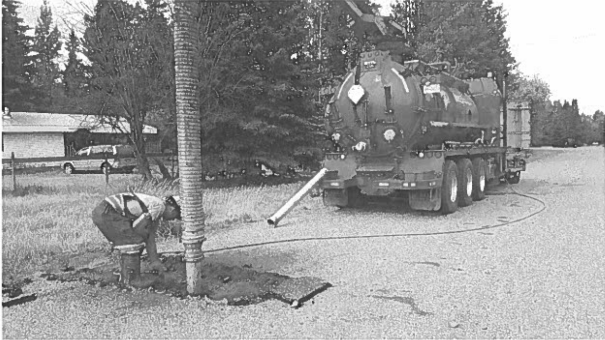
FIGURE 10 – VAC TRUCK EXPOSING EXISTING WATERMAIN TO DETERMINE TYPE AND LOCATION
