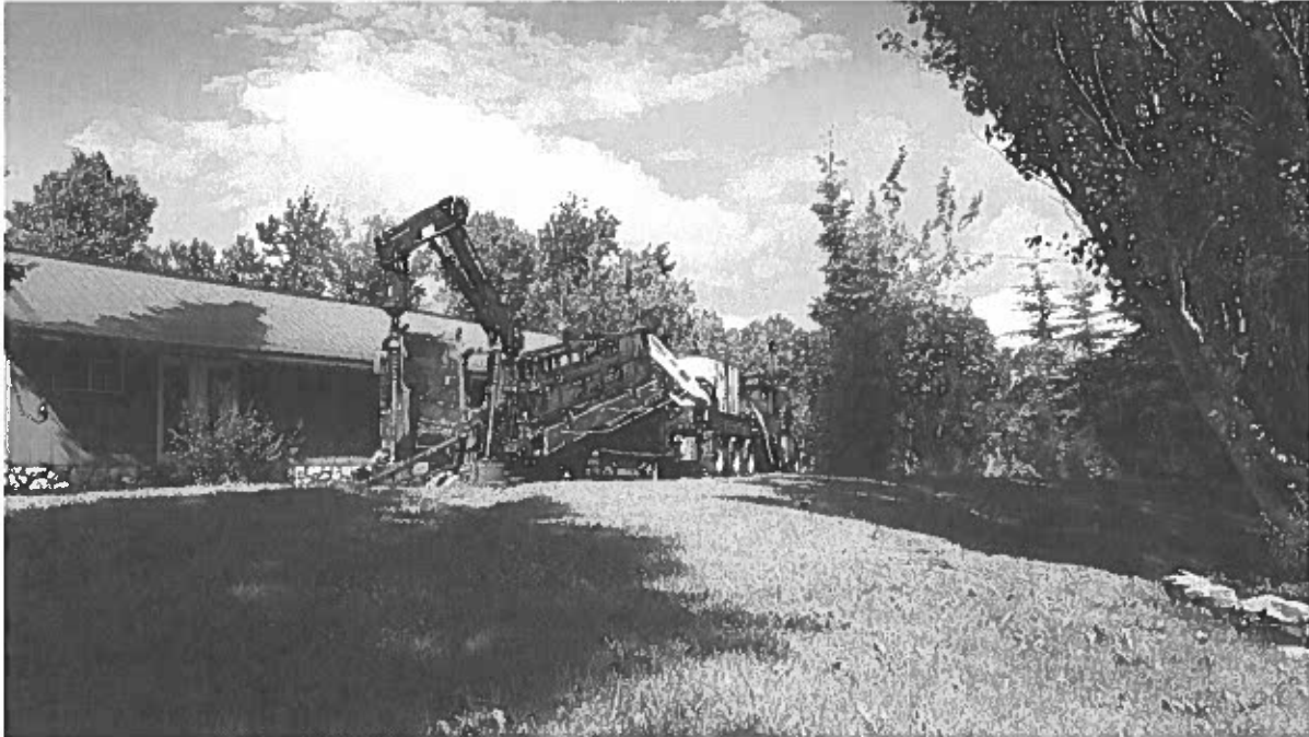
FIGURE 3 – DRILL RIG SET UP FOR CORPORATION STREET LONG SERVICE
