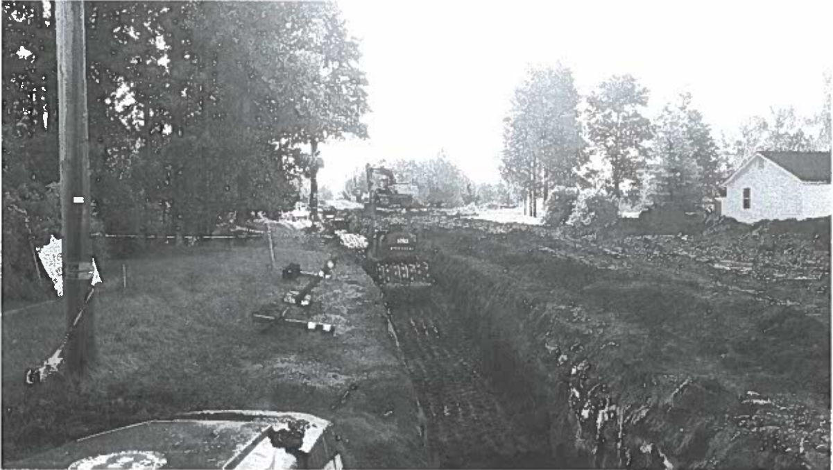
Backfill Crew Continuing to Work on 5 th Avenue
