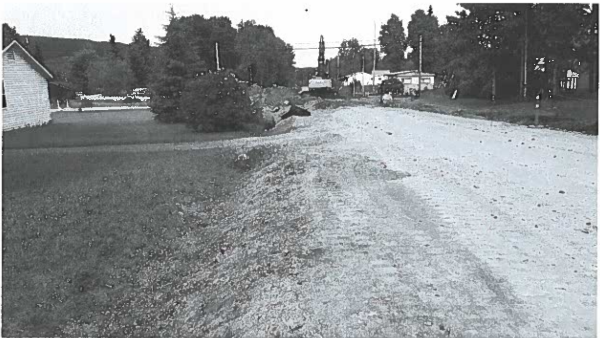
5 th Avenue South Ditch Restored to Original Condition
