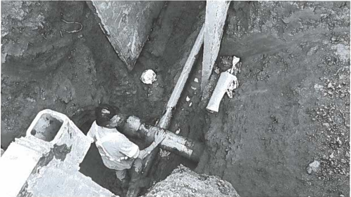
Shrink Wrap on Both the Sanitary Sewer and New Watermain Joints
