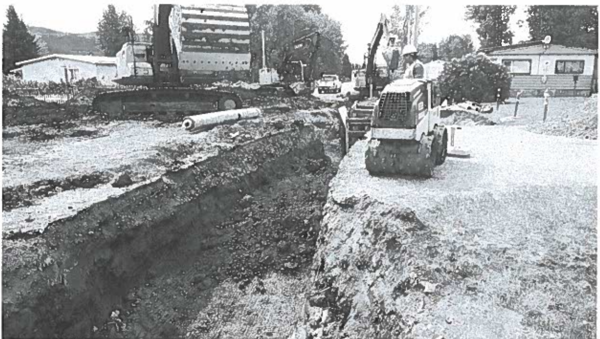
Geogrid and Out-sourced Drier Backfill Material Placed in Corporation St Crossing
