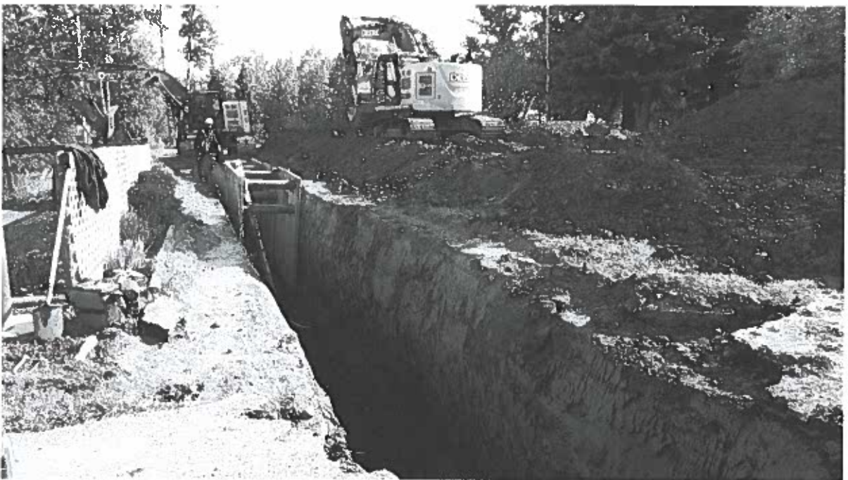
Pipe Crew on Corporation Street Near the Fire Hall
