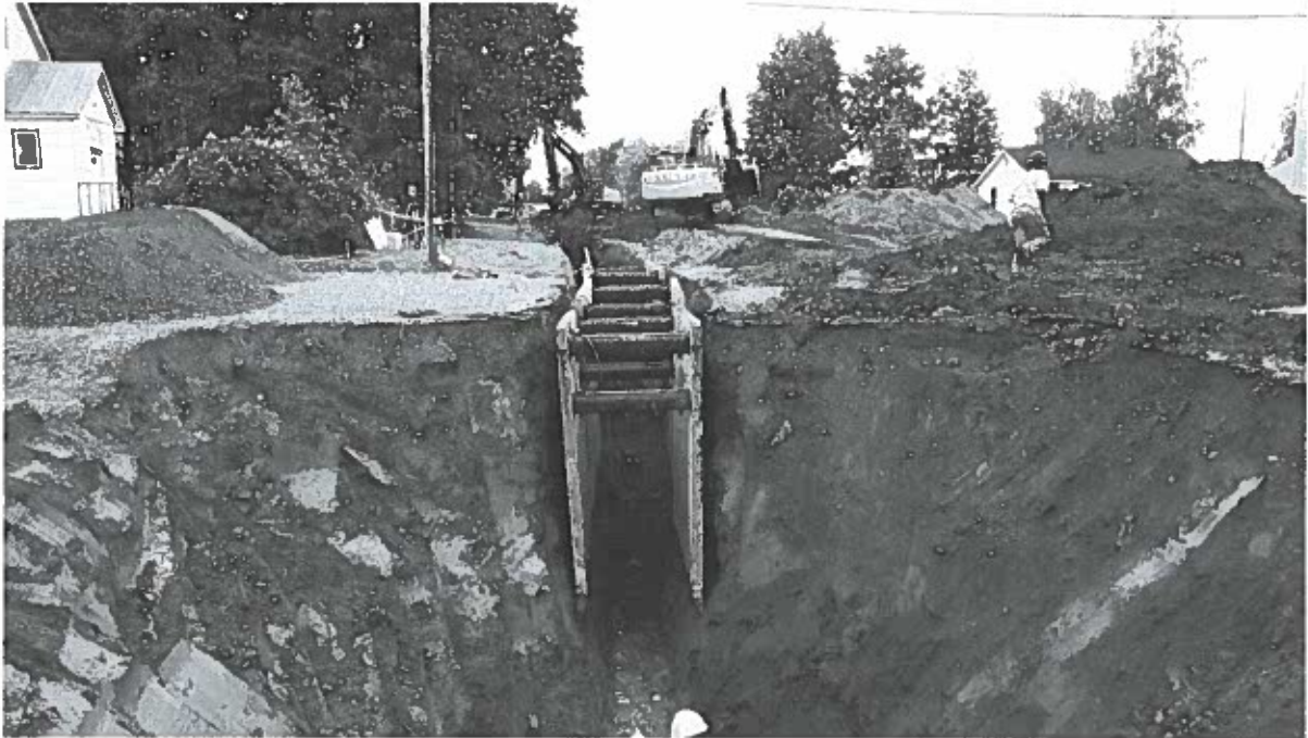
Pipe Crew Crossing Corporation Street
