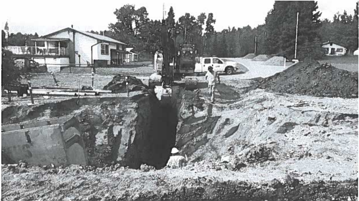
Pipe Crew Starting on Corporation Street (North)
