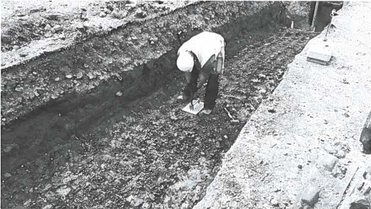
GeoNorth Engineering On Site Testing Compaction in the Road Crossings
