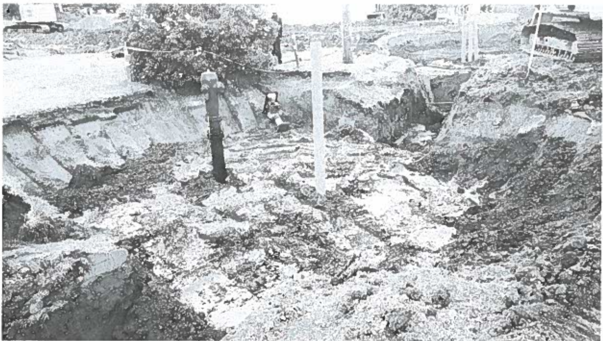
Fire Hydrant Installed on 5 th Avenue at Approx. Sta 0+720m
