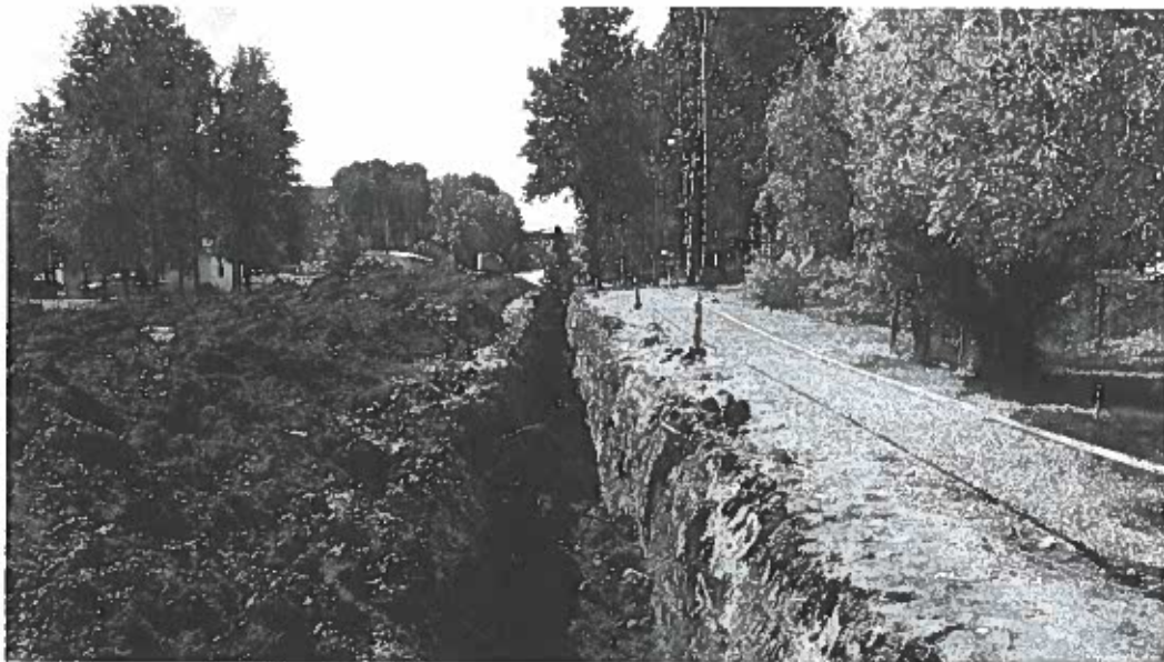
Open Excavation on 5 th Avenue
