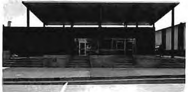
SILGA – Southern Interior Local Government Association: Town of Summerland for the R.C.M.P. Building
