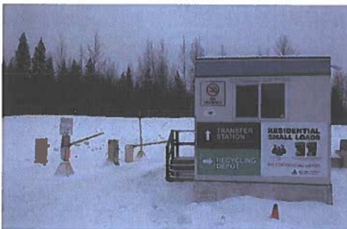
Figure 3-5: Regional District of Fraser Fort-George Vanway Transfer Station
