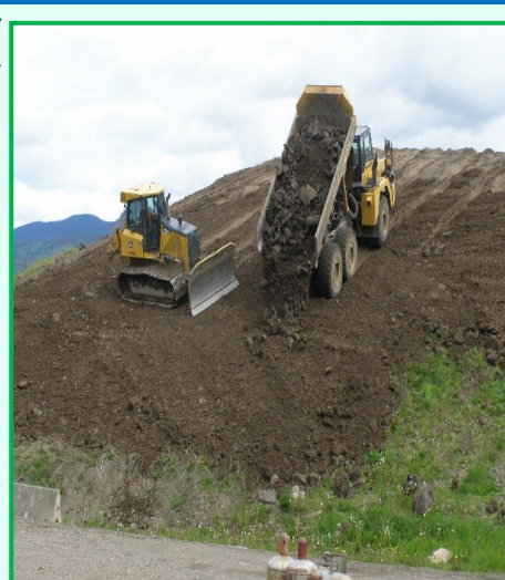
(Equipment working on covering the landfill)
