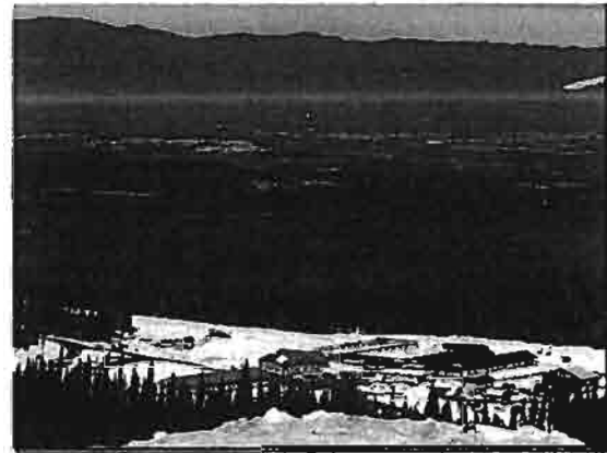
Photo ES 27: Blackwater Exploration Camp
