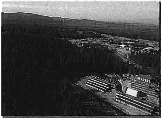
Photo ES 33: Blackwater Exploration Camp
