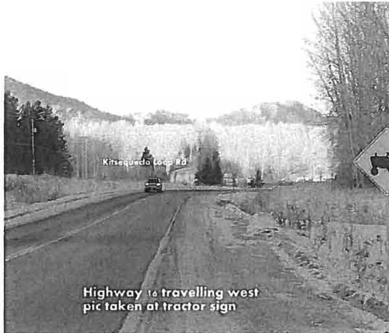
Photograph 4: Highway 16 looking West
