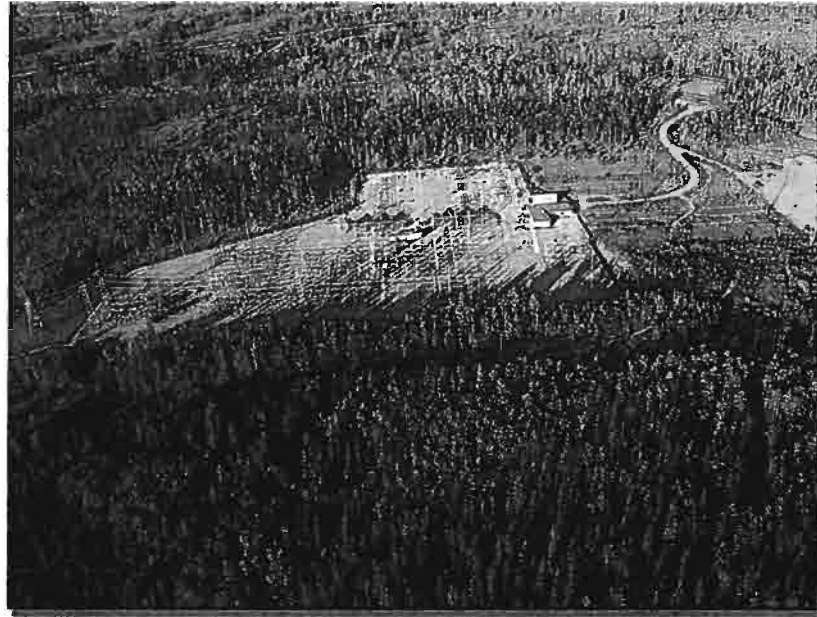
Photo ES 2: Aerial View of BC Hydro Substation, south of Endako
