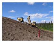
Final closure works at the old Burns Lake Landfill were completed including the establishment of suitable grading, placement and compaction of low permeability soils on previously landfilled areas, and grass seeding. Work to update the Environmental Moni-
